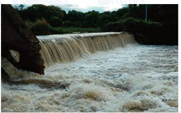
Water flowing over a dam creates a dangerous backwash current known as hydraulic suction.
