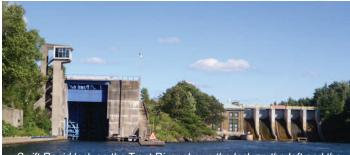
Swift Rapid lock on the Trent River shows the lock on the left and the dam on the right
